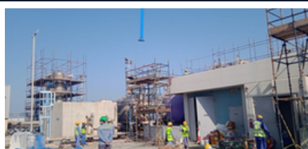
Steel Structural Works- DEWA
