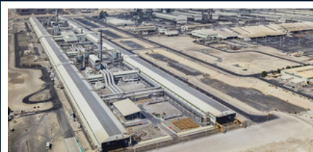
Casthouse Extension- EGA
