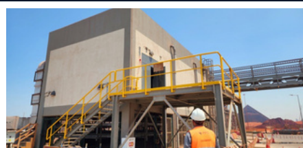
OBxR Sub Station Works- ATA
