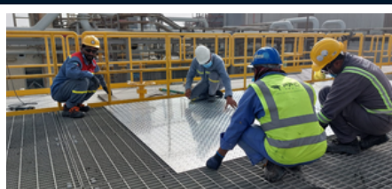
Repair & Replacement of Batch Homo & Circuit- EGA
