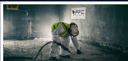
Curtain Injection Works- Gulf Extrusions
