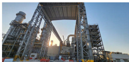
700T Structural Crane- EGA
