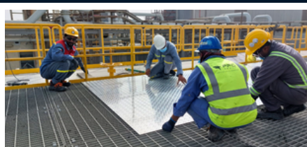
Steel Structure Repair & Replacement- DP WORLD
