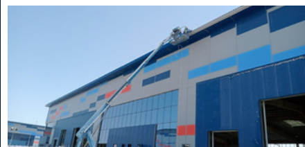
Critical Warehouse Storage Phase 1- KEZAD
