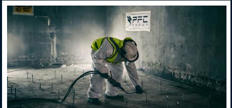
Curtain Injection Works- Gulf Extrusions
