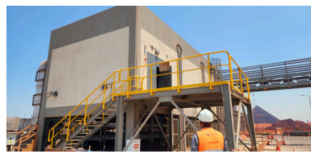
OBxR Sub Station Works- ATA
