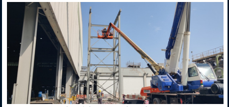
Industrial Structural Works- EGA
