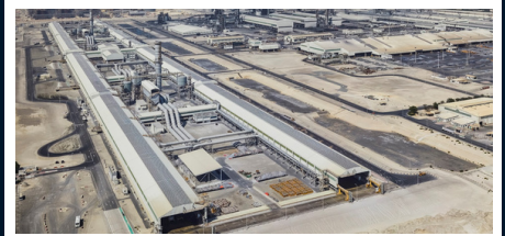
Casthouse Extension- EGA
