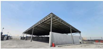
Storage Facility- EGA
