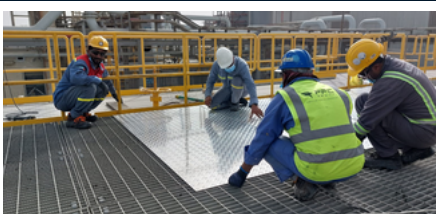
Repair & Replacement of Batch Homo & Circuit- EGA
