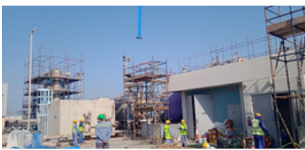
Steel Structural Works- DEWA
